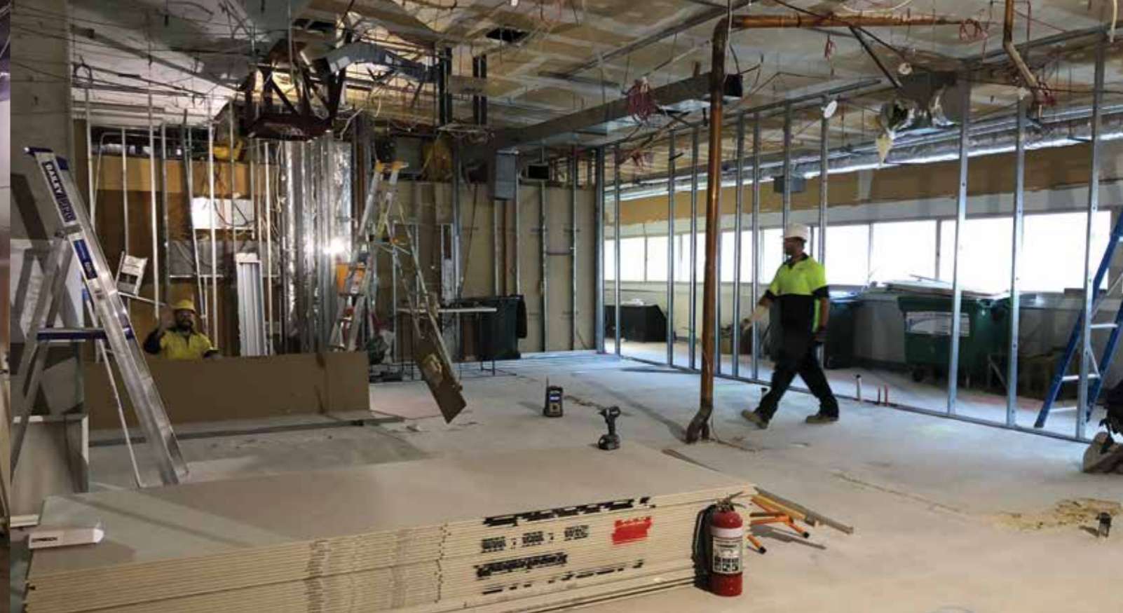
Raelee Denniston and GM Claire Fogarty check on the construction progress
